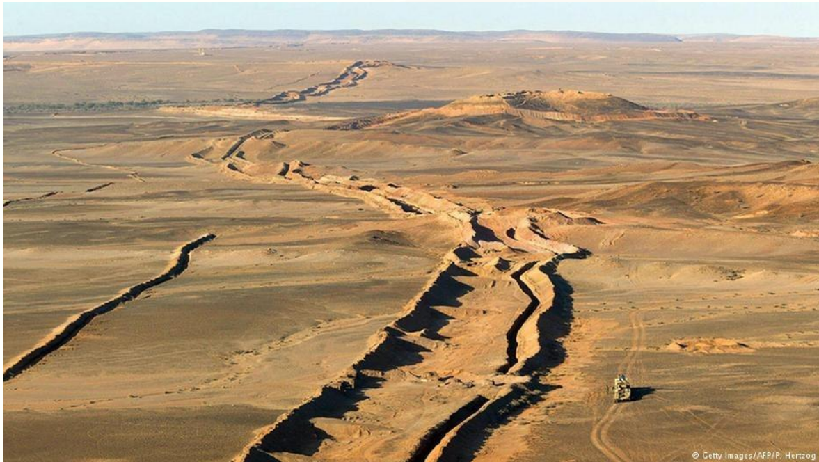
Figure 4 : Image of the Berm.
